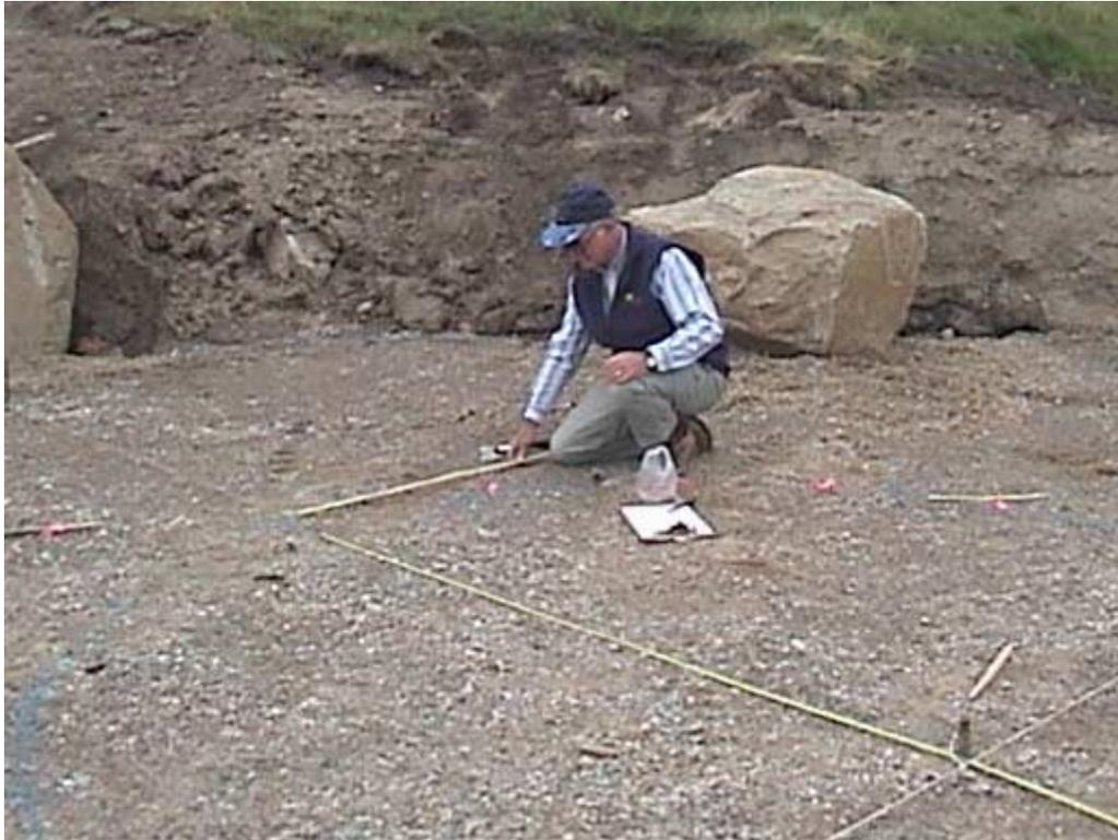
Roger Bailey is shown above establishing the position of the hour markers according to the data from the design spreadsheet and the drawing shown below.
