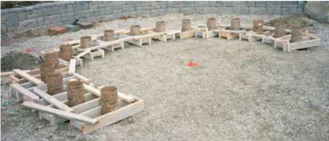
The bronze plaques, horseshoes and sun were set into the Zodiac Table that was precast in separate pours for each colour. Three separate concrete pours were required for the posts, the hour ellipse and the final base. The bronze numbers, plaques and horseshoes were cast in as the concrete was poured.
